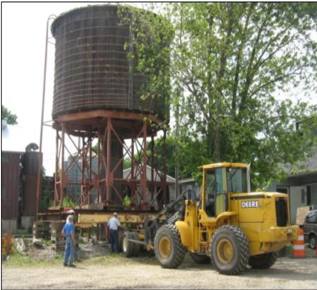
Water Tower Relocation 2008
